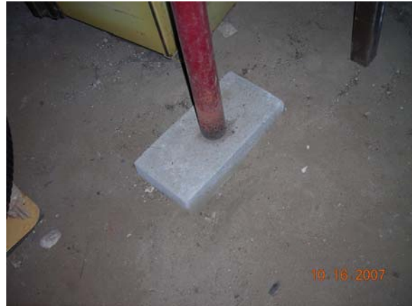
Photo 8 Concrete Block Footing
