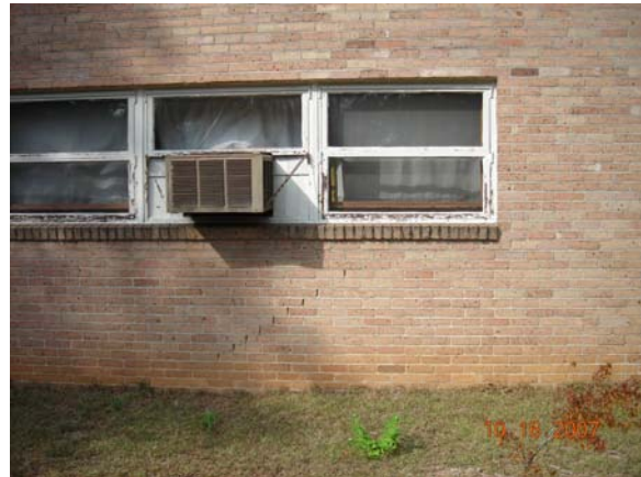
Photo 2 Veneer Cracks
