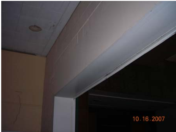
Photo 1 Roof Leaks
